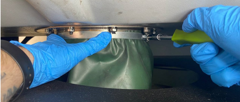
Figure 21. Mounting the drain collar
