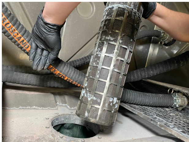
Figure 46. Removed tank filter
